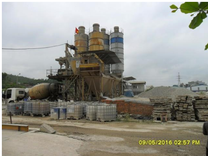
(Piling and starting the construction)
